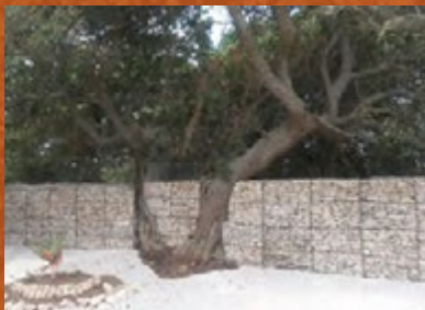
Carl Gous(Gabion Baskets) – 082-8203883 – WC
